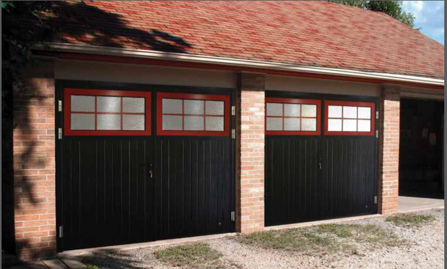
Glazing panels in contrasting 'Flame red' colour.
